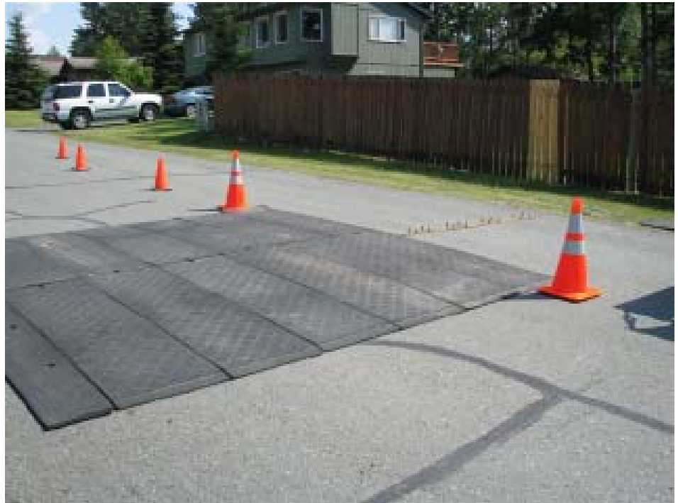
Speed bump installation underway in an attempt to curb speeding motorists.
