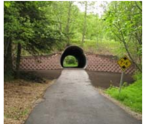
Completed retaining wall
