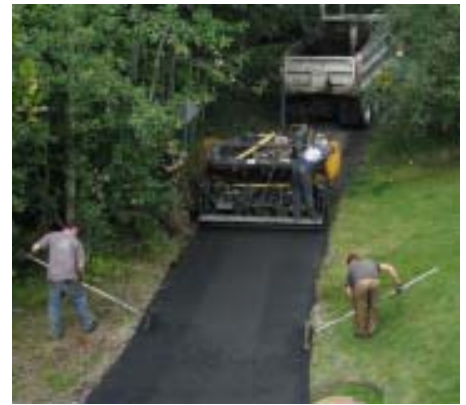
New trail replacement in process
