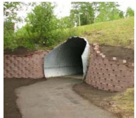
Another retaining wall finished
